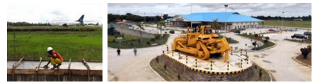
Mikmika Airport drainase
