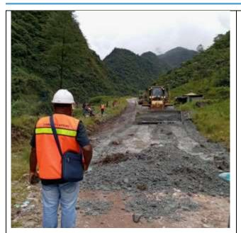
The process of revitalizing the main road access to Waa Banti village using *gravel* sand taken from the CIP 72 area of PTFI.
