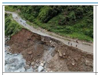
Increased water flow rate in the river resulting from high rainfall damaged river embankments, disrupting access to the main road from Tembagapura to Kampung Waa Banti.
