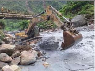
The normalization process for Agawagong River to prevent erosion of retaining structures supporting bridges in Kampung Waa Banti.
